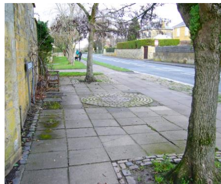
Well-paved footpaths and sett-lined kerb finishes
