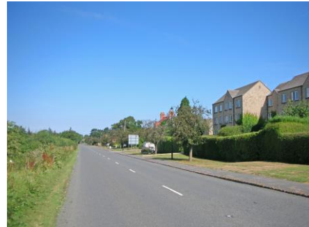
Station Road looking west
