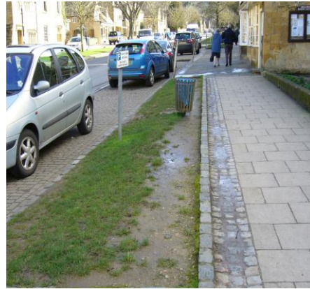
Poor maintenance of grass verges
